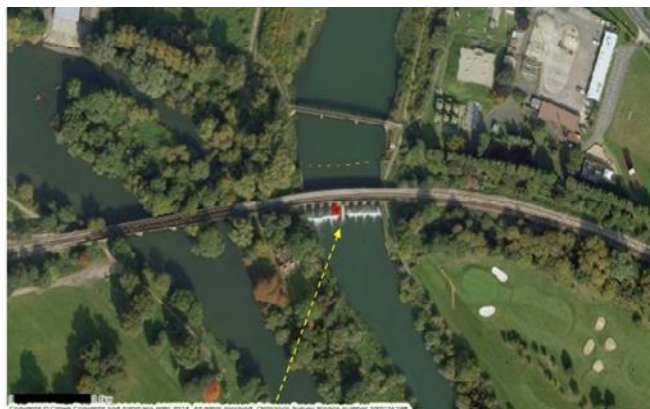
Aerial view of Black Potts weir
