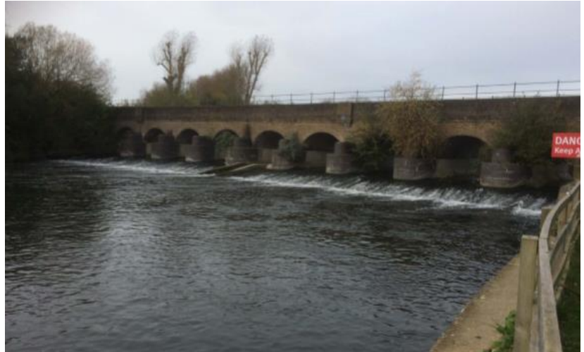
View of Black Potts weir, looking upstream
